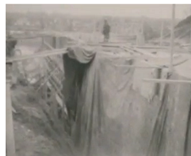
Figure 1.3: Steam tunnels being built for heating in the 1920s.
