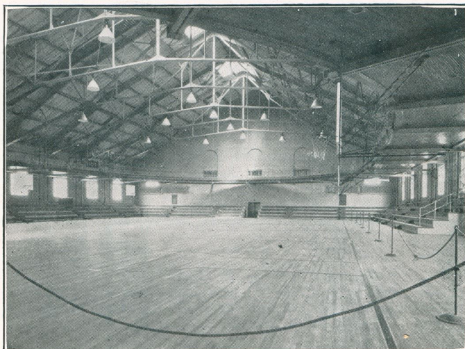
MAIN GYMNASIUM ROOM, BROWN UNIVERSITY GYMNASIUM
