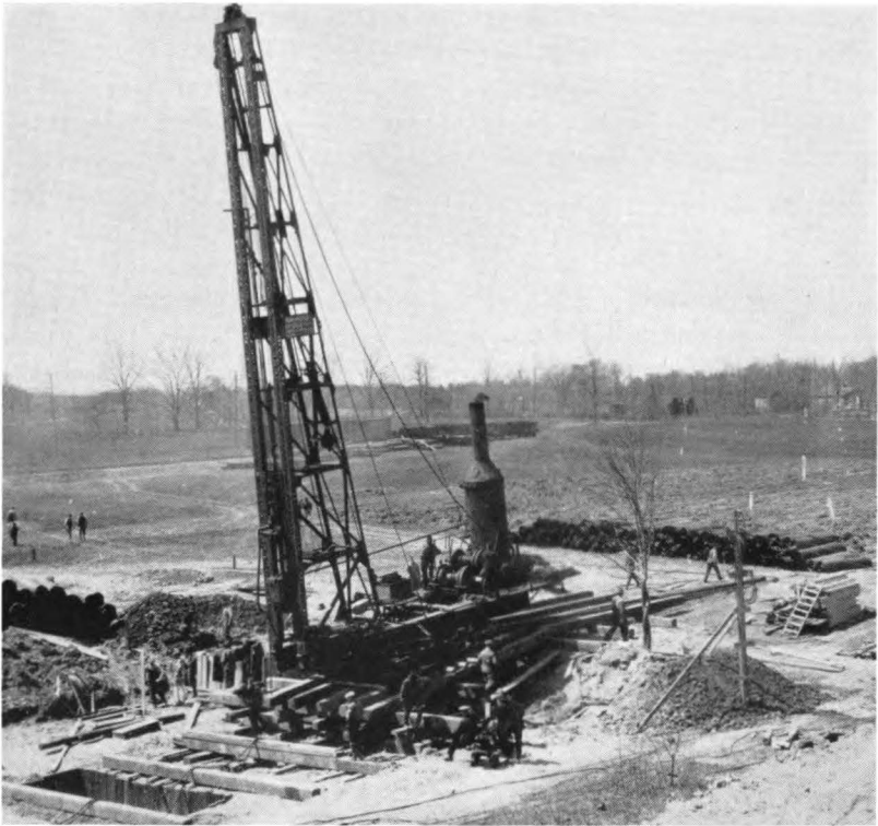
Pile driver moves into excavation of main building. In the background to the south is the Lehigh Valley Railroad spur which then ran parallel to the trolley tracks in Crittenden Boulevard.
