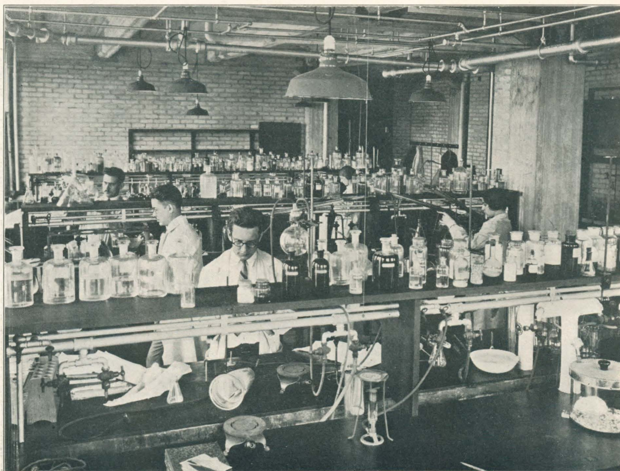
FIG. 3.—ADVANCED STUDENTS' LABORATORY SHOWING ARRANGEMENT OF SHELVING, SUPPLY PIPING, AND DRAINS
