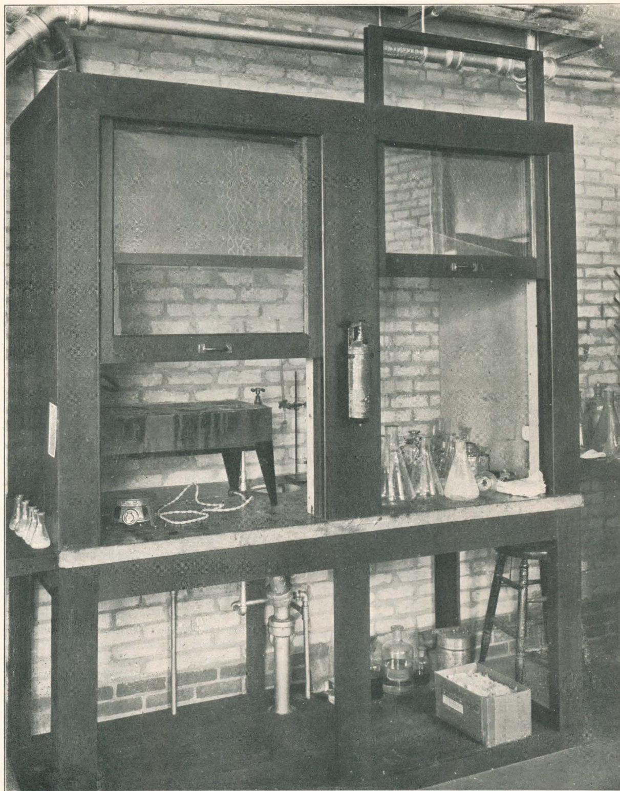
FIG. 1.—FUME-HOOD. TYPE USED IN MOST LABORATORIES THROUGHOUT THE BUILDING
