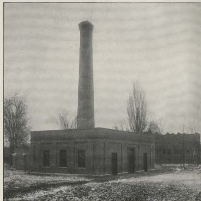
CENTRAL HEATING PLANT
