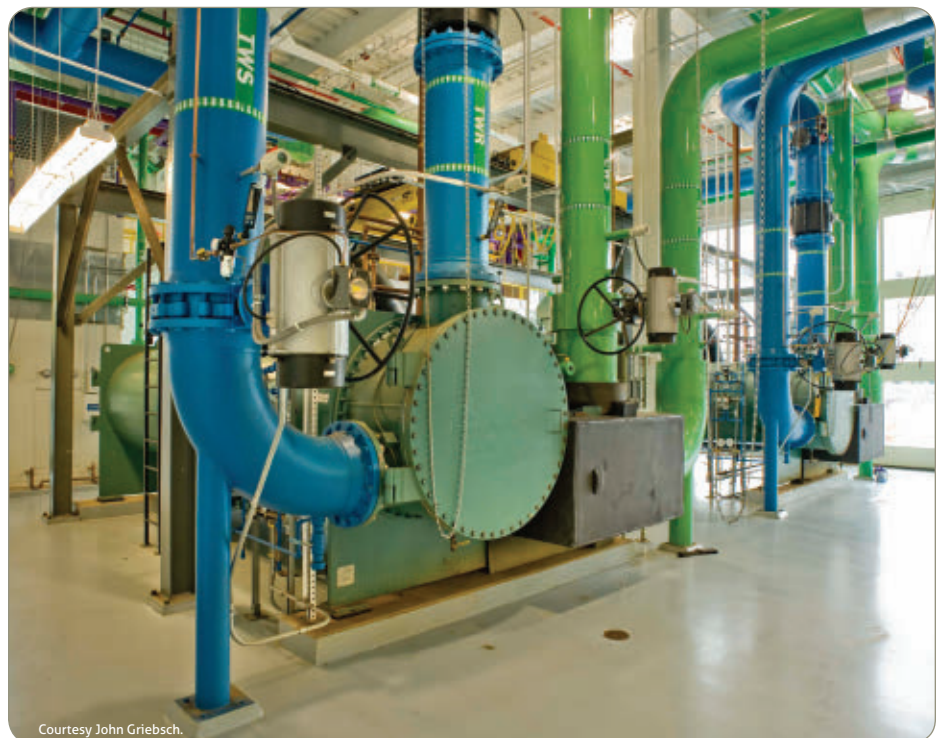
View of chillers No. 6 and No. 7 within the MCCP.
