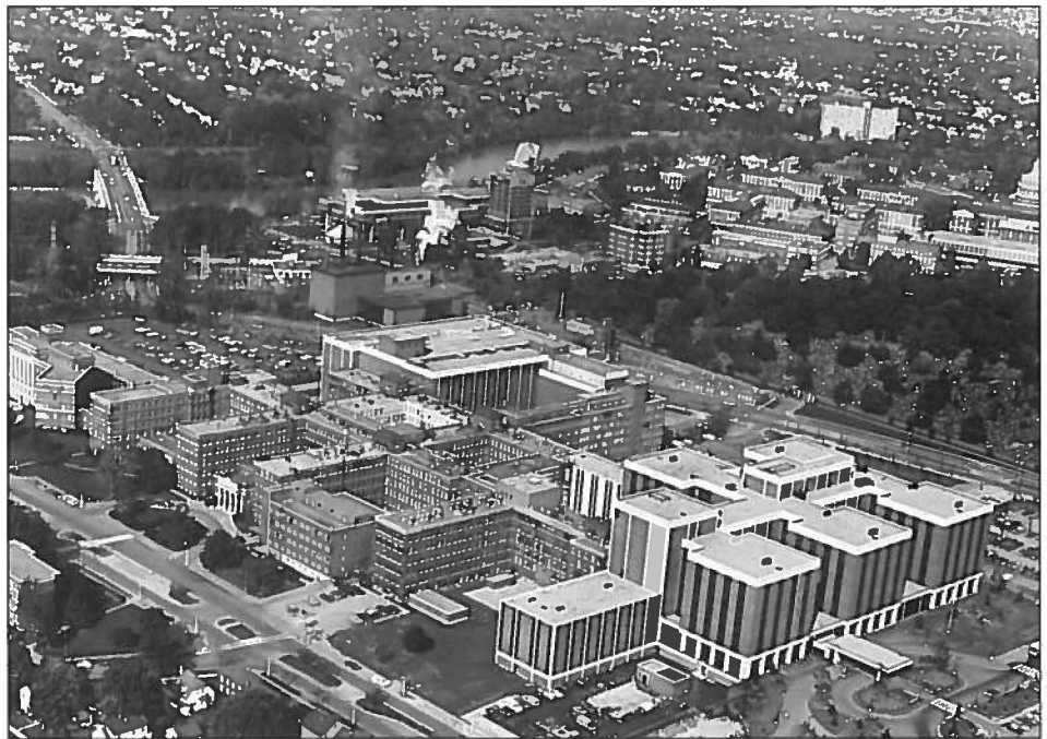
The University of Rochester's Central Utilities Plant (upper left) serves both steam and chilled water to campus buildings.
