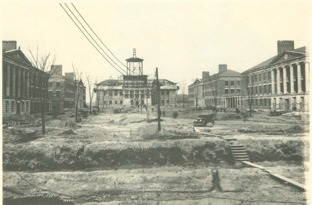
The Quadrangle is under construction in this photograph from April of 1929. From 1927 until the fall of 1930, a total of 11 buildings on the original campus were completed.
